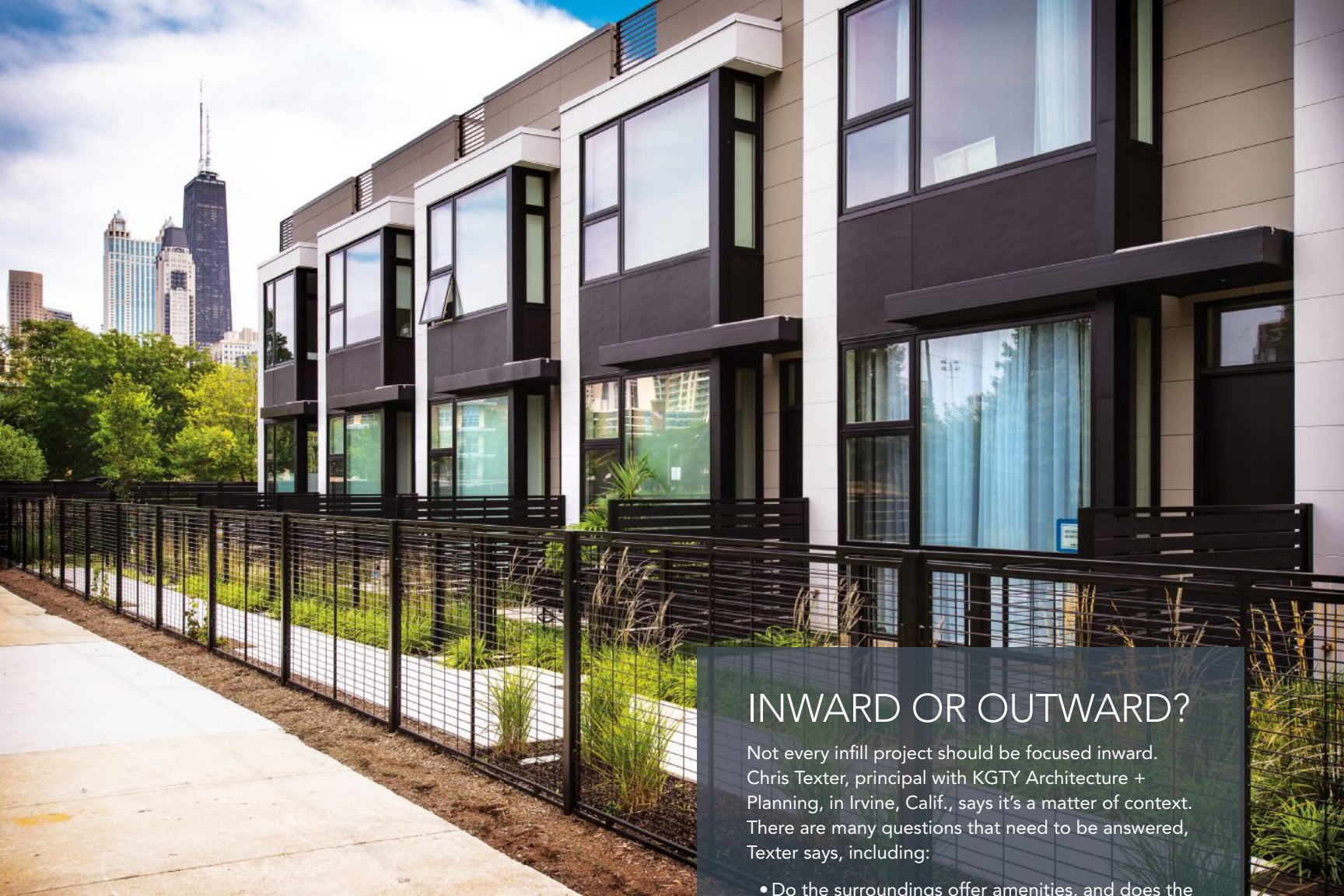
THE LOW-RISE BUILDINGS OF BASECAMP RIVER NORTH OFFER A STRIKING CONTRAST TO NEARBY HIGH-RISE BUILDINGS, INCLUDING CHICAGO'S FAMED JOHN HANCOCK TOWER.
